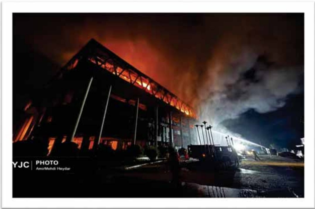
Iran State TV Building on Fire, during attacks on 16 June 2025
